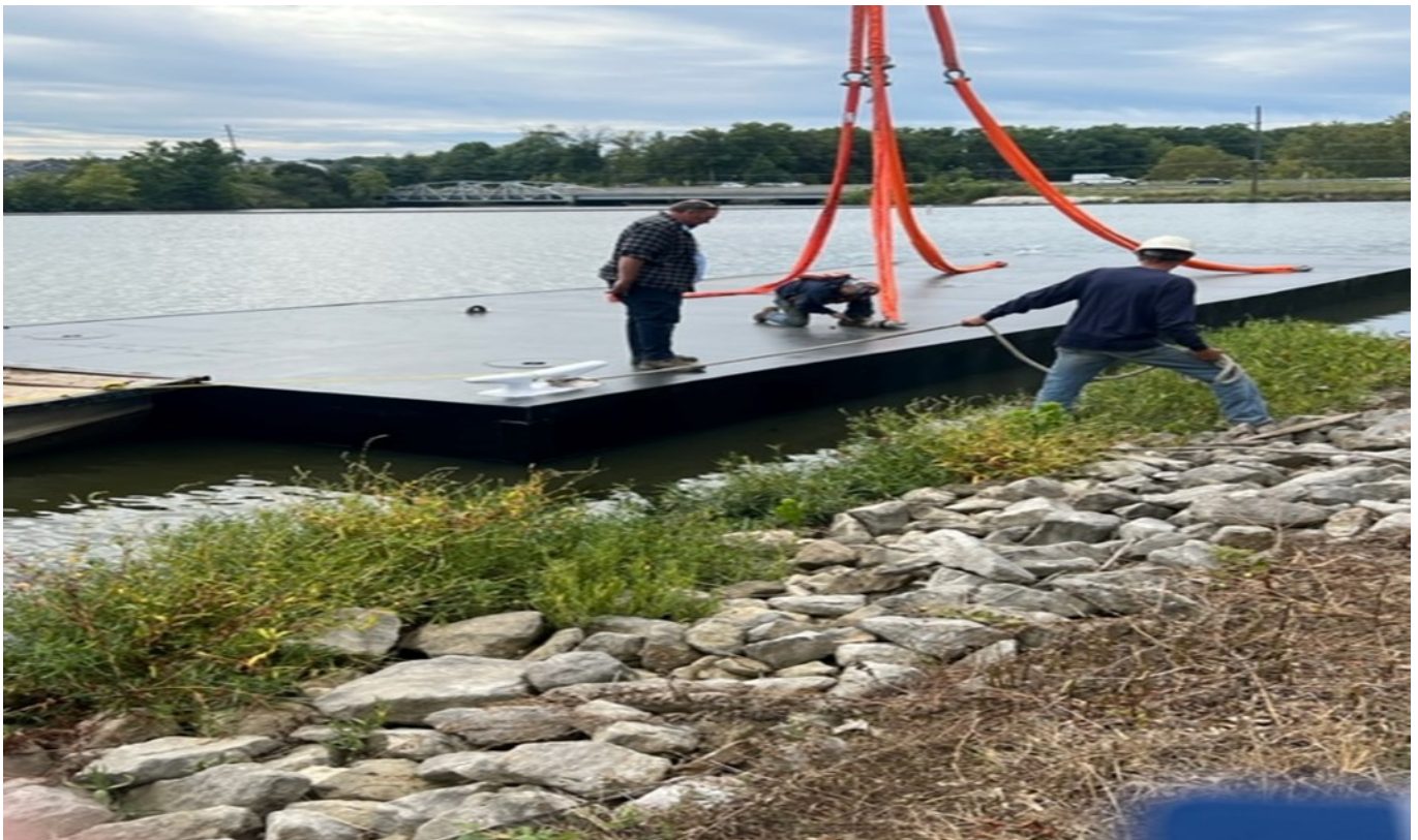
(New Work Barge)
